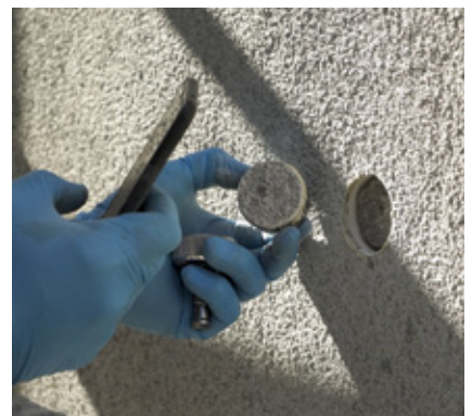
Adhesion tensile test of the MC-RIM mortar coating
